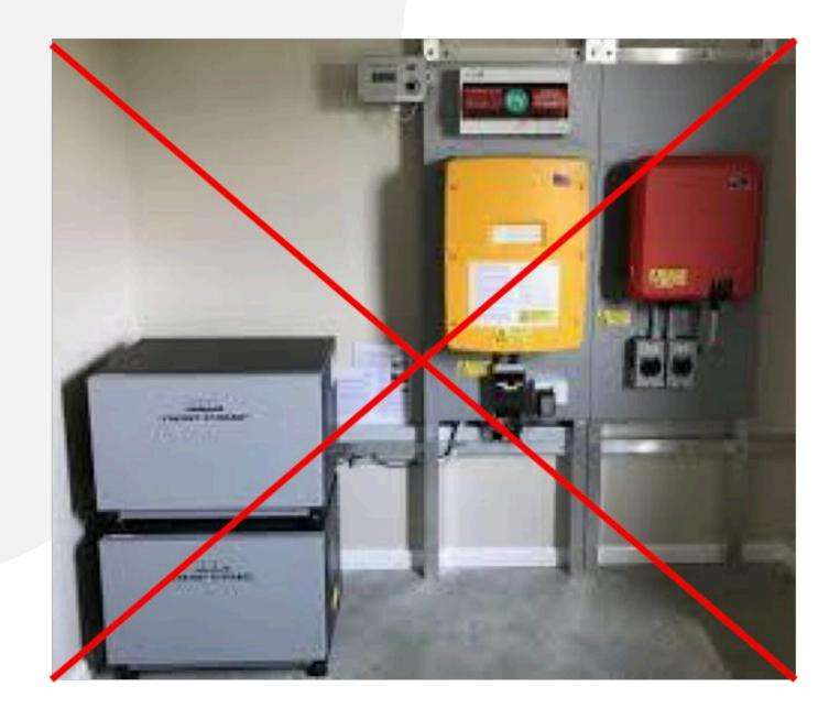
Solar Charge Controller Grid Inverter Battery Bank
